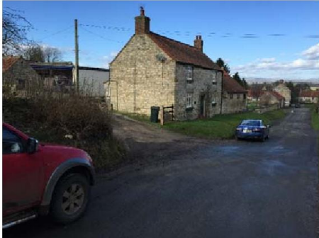
Existing access next to Smiths Cottage
