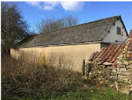
Existing abattoir buildings from outside site
