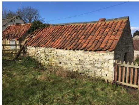
Existing abattoir buildings from outside site
